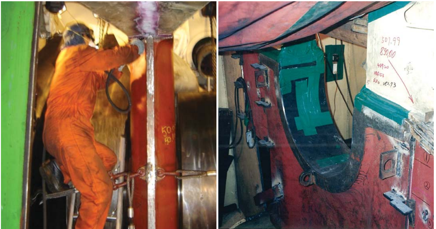
▲ Replacement of main bearing saddle (Girder)
